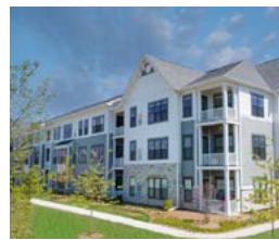
Stacked Flats Example: The Sixteen30 in Plainfield, IL
