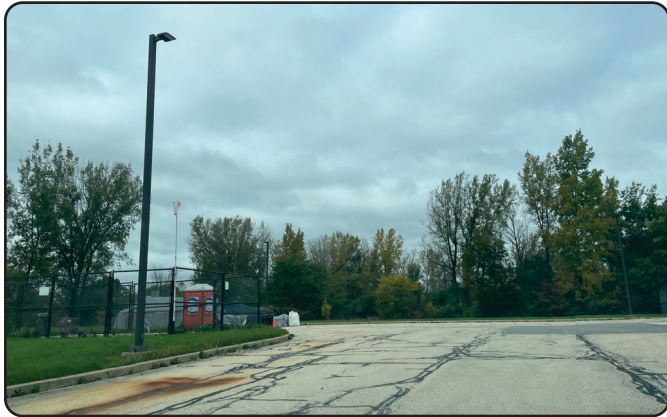
(3) LED pole fixtures, as well as their drivers and fuses, to be replaced at the Water Treatment Facility
