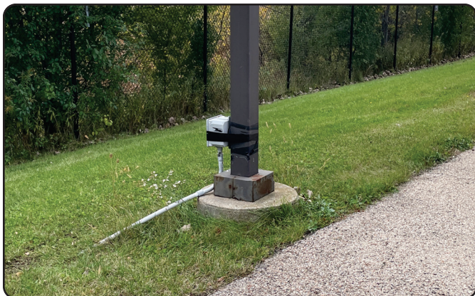
O'Carroll to clean up this pole base stub-up
