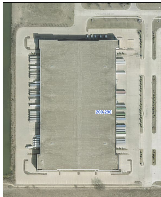
Figure 1: GIS Snapshot of the Sub Zero Group Building
