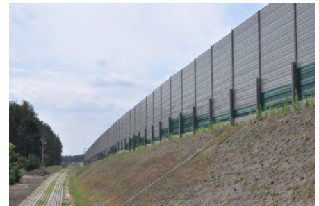
REAR-VIEW OF HIGHWAY BARRIER
